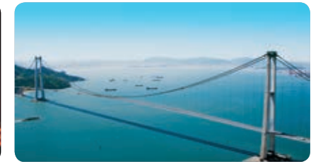
Suspension Bridge (Yi Sun-sin Bridge)
