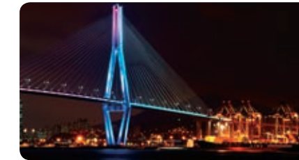
Cable Stayed Bridge (Busan Harbor Bridge)
